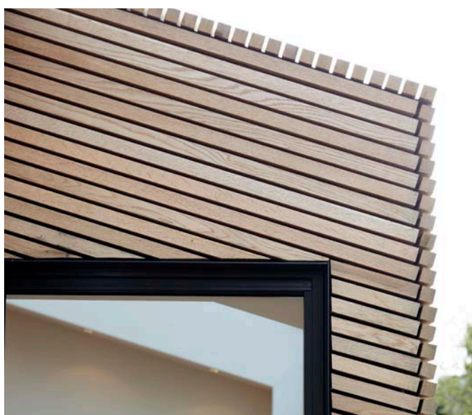
American white oak, used for the external cladding of Church Crescent house by Evonort Architects.
